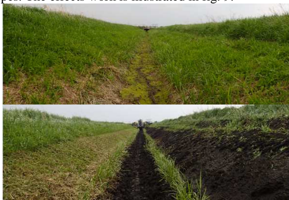
Fig. 9. Condition of watercourse; the photo at the top shows a ditch before desilting, the photo below shows a ditch after desilting while mowing grass on slopes
